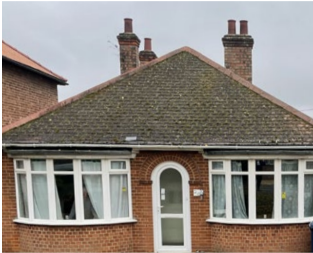
BAY WINDOWS; CHIMNEYS
