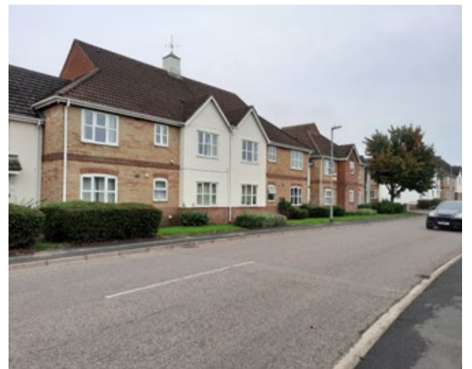
LOW HEDGES AND SOFT LANDSCAPING TO THE FRONT OF DWELLINGS AT QUIETER STREETS
