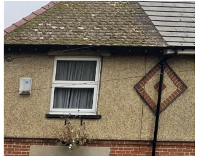
DECORATIVE BRICK DETAILING
