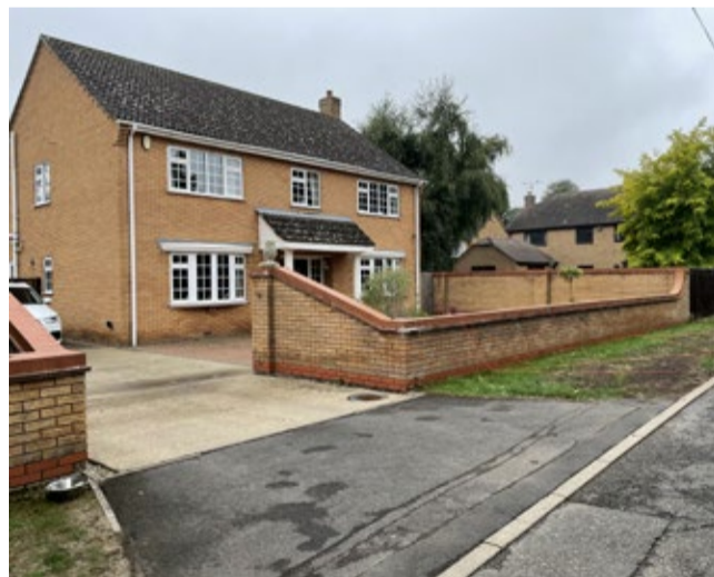
BRICK WALL AS BOUNDARY TREATMENT
